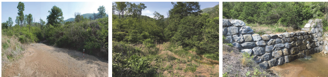
Fig. 7. View of Filled Erosion Control Dam in Forestfire-Damaged.
