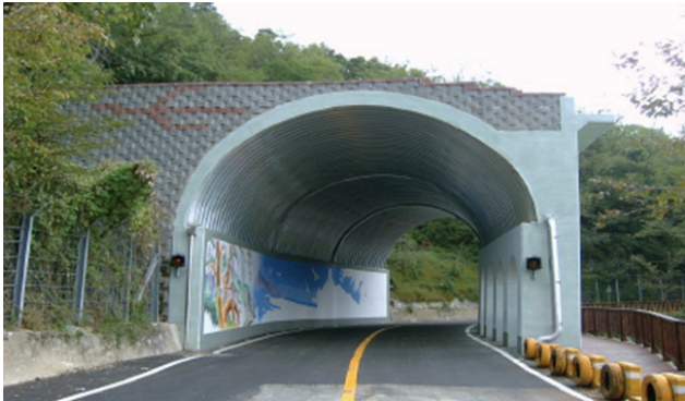
Fig. 1. Corrugated Steel Plate Tunnel
