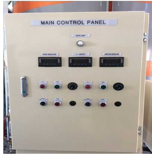
(b) control panel of mixer
