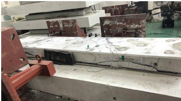
Fig. 8. Crack Shape of Specimen Loaded at Center Point
