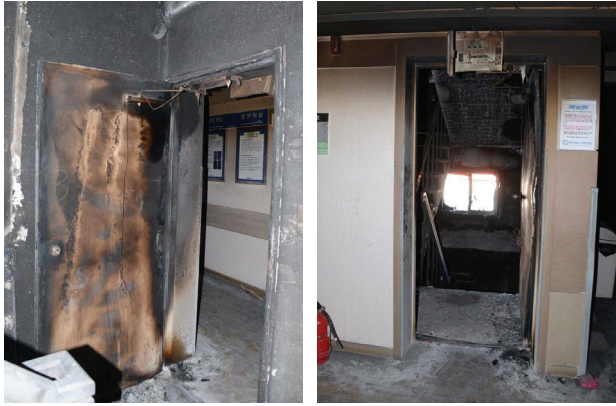
Fig. 12. Around Main Fire Door on the 3th Floor
