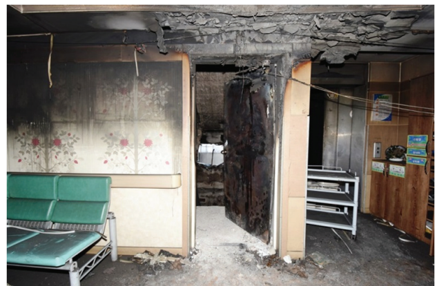
Fig. 11. Around the Main Fire Door on the 2nd Floor
