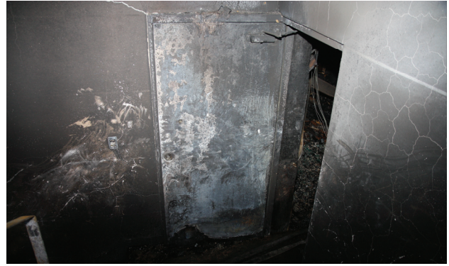
Fig. 9. Fire door of Main Entrance in the 3th Floor
