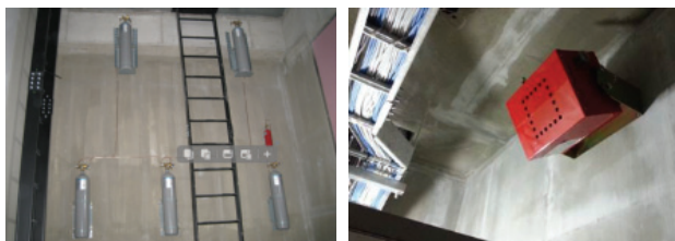
Fig. 5. Small Space Automatic Fire Extinguisher
