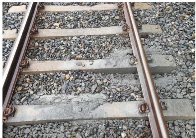
Fig. 6. Mud-pumping Occurrence
