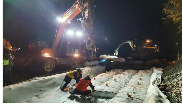
Fig. 4. Construction Site Being Installed
