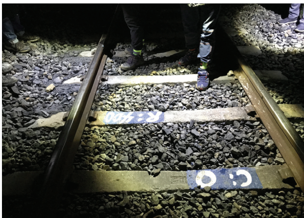
Fig. 5. Settlement of Sleeper
